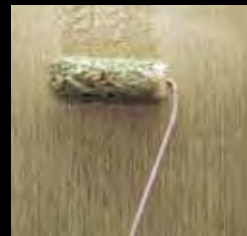
applicare 2° strato di creative ard sand gold o silver apply the second layer of creative ard sand gold or silver
