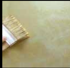
applicare 2° strato di creative ard sand gold apply the second layer of creative ard sand gold
