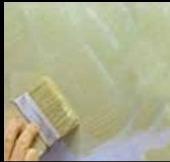
applicare 1° strato di creative ard sand gold apply the first layer of creative ard sand gold
