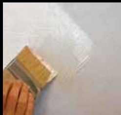
applicare 1° strato di creative ard sand silver apply the first layer of creative ard sand silver
