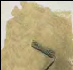
applicare 1° strato di creative ard sand gold o silver apply the first layer of creative ard sand gold or silver
