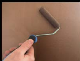
applicare 2 strati di creative ardcopper-base apply 2 layers of creative ardcopper-base
