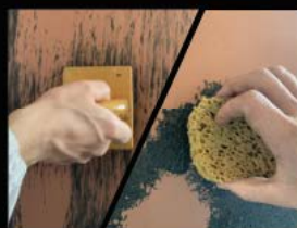
applicare creative ardrust-base con zerbino o spugna marina apply creative ardrust-base with sea sponge or plastic brush
