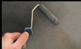
applicare 2 strati di creative ardrust-base apply 2 layers of creative ardrust-base
